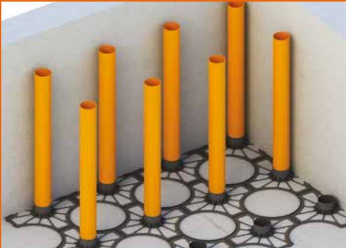
Place the tubes in PVC in the base grids and lock them pushing at the top of the tubes.
