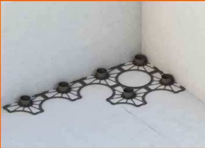
Cut the base as in the picture and place the first row against the wall, starting from the right.
