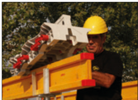
① PLACE OF THE Y BEAMS + WEDGE
