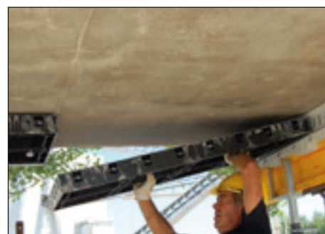
⑨ REMOVAL OF THE GEO-PANEL PANELS
