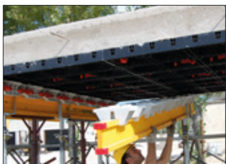
⑦ REMOVAL OF H BEAM
