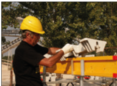
② PLACE OF THE H BEAMS
