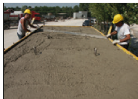
⑥ CONCRETE LEVEL-LING
